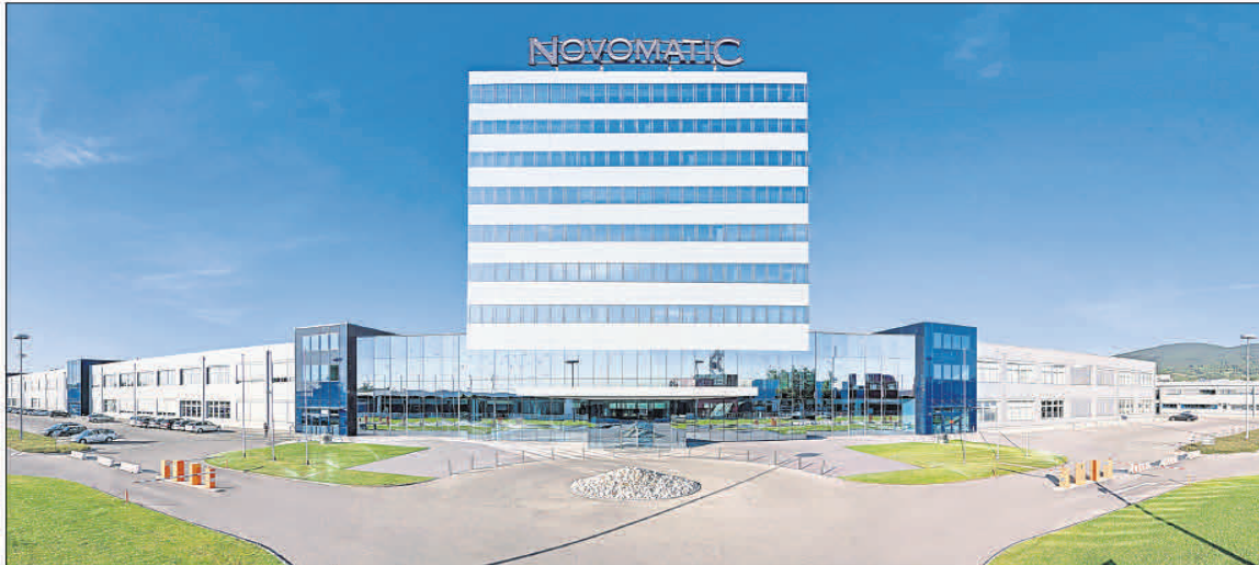
Novomatic-Headquarter in Gumpoldskirchen, Niederösterreich.
