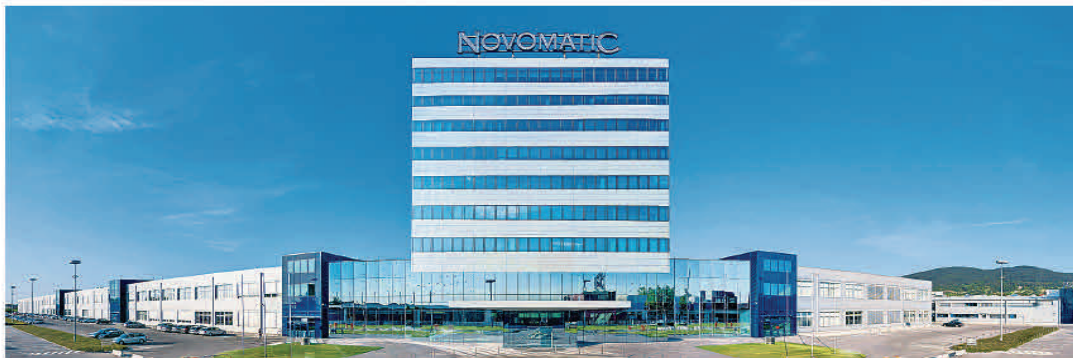
NOVOMATIC-Headquarter in Gumpoldskirchen, Niederösterreich
