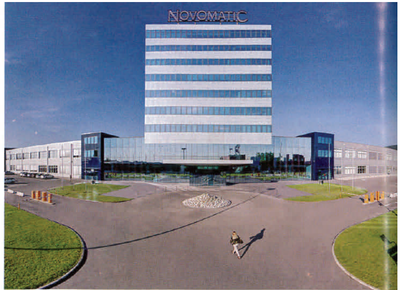
Novomatic Headquarters, Austria
