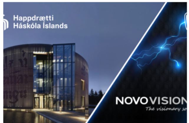
The University of Iceland Lottery has installed NovoVision
